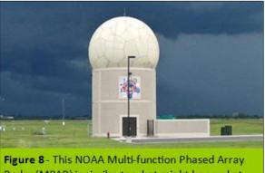
Figure 8 - This NOAA Multi-function Phased Array Radar (MPAR) is similar to what might be used at Boca Chica. It is designed to provide aircraft tracking as well as wind profiling and weather surveillance.
